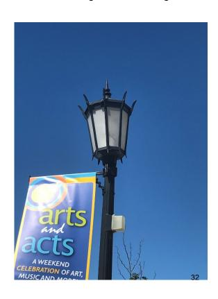
This year, the DDA will be replacing roughly 100 lights from Hight Pressure Sodium to LED. The DDA spent a lot of time selecting the LED light source which is the most compatible with the existing Induction Lighting. The LED light that was selected was a 2700k warm white light. The LED lights will be retrofitted in the Herwig luminaries and will provide a substantial cost savings over buying all new luminaries.
